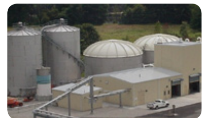
Distillery, Puerto Rico Biothane Biobed® Advanced UASB
