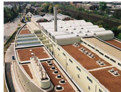
Herford, Germany (1997) - 250 000 PE Nitrification/denitrification after physical-chemical settling. 4 cells, 63 m 2 each
