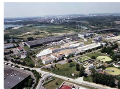
Saint-Thibault-des-Vignes, France (2000) Post-denitrification after nitrification/denitrification. 4 cells, 63 m 2 each 350 000 PE
