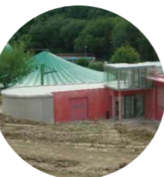
Douarnenez, France (2003) Post-denitrification after nitrification/denitrification. 5 + 1 cells, 63 + 28 m 2 each 80 000 PE
